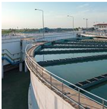
Tap water plant
